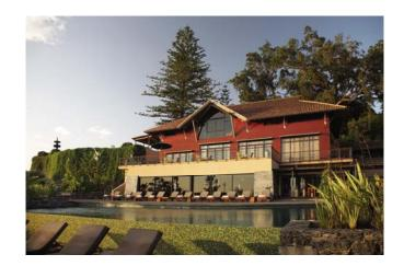
b. <u>Roof.</u> The height of a building and the type of roof design significantly influence the scale of a building. Roofs shall generally be of a gable or other sloping roof design. Roofs shall have a minimum pitch of 7:12. Roof lines shall be integrated into the facade and structure of the building and use of any kind of a parapet to simulate a roof line shall be prohibited. [This is the fake mansard or other roof prohibition]
